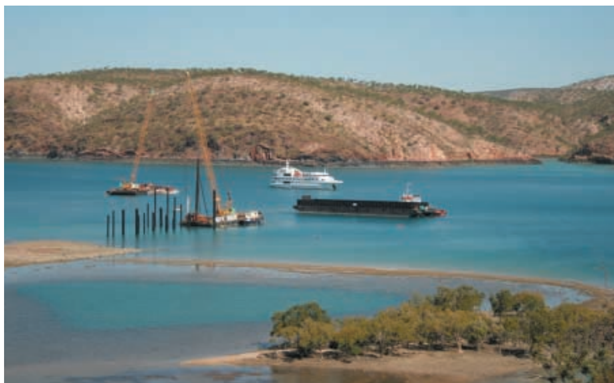
From Construction to Production: Almost 50% of the jetty piling is complete on Koolan Island.
