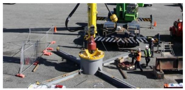
The SRP designed CETO 5 connector (red component in centre) during onshore testing, 2015
