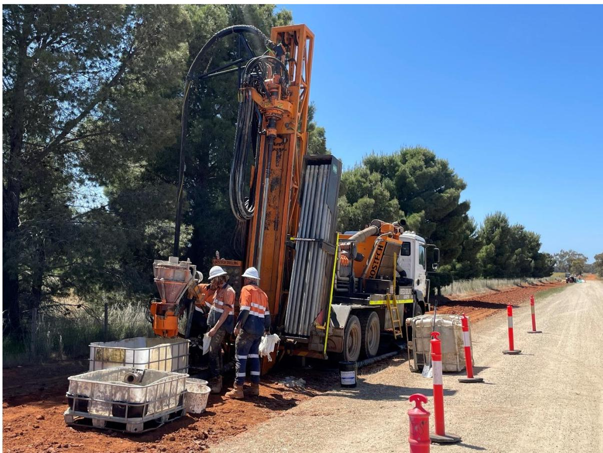
**Figure 2** Aircore Rig drilling for mineral sands and REE at the Pyramid Hill Project
