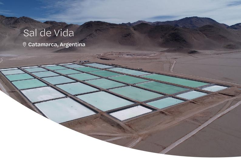
Sal de Vida is designed to produce battery grade lithium carbonate through an evaporation and processing operation located in Catamarca Province, Argentina, approximately 200km from Olaroz. The Feasibility Study for this wholly owned project focuses on an initial 11ktpa operation that can readily expand to ~32ktpa through later stages.
