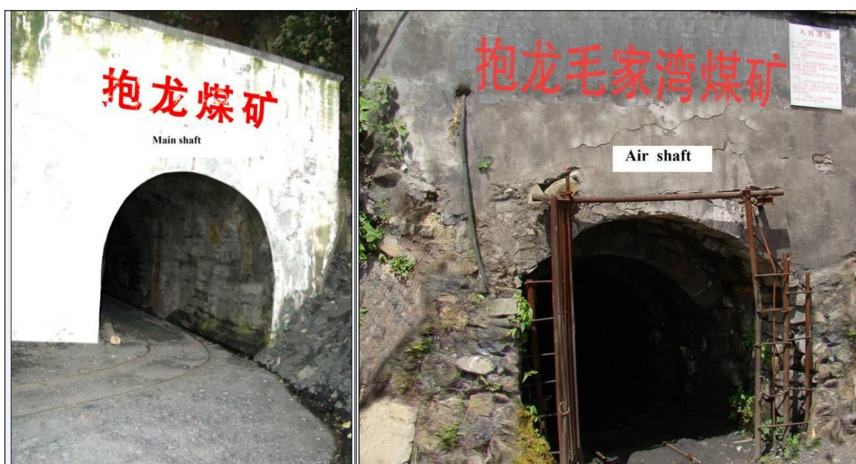
Plate 3: Baolong Maojiawan No 1 East Mine Production Adit (L) and Ventilation Adit (R).
