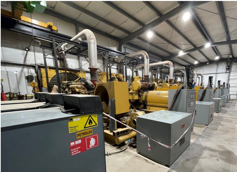
Disconnected backup Power Grid (6 x 1MW diesel Gensets)
