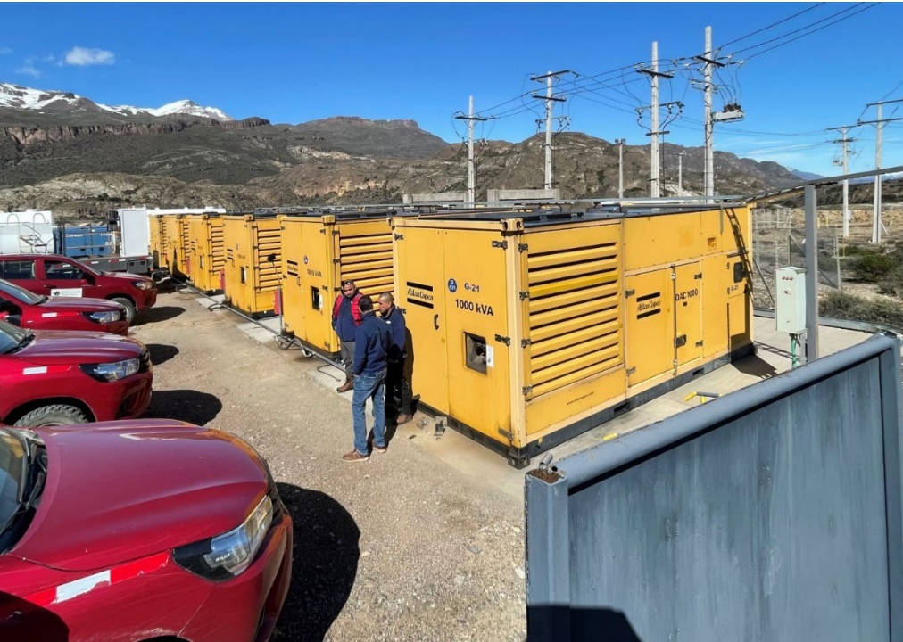
Current Power Grid (6 x 1MW installed + 3 spare + 1 x 500KW)
