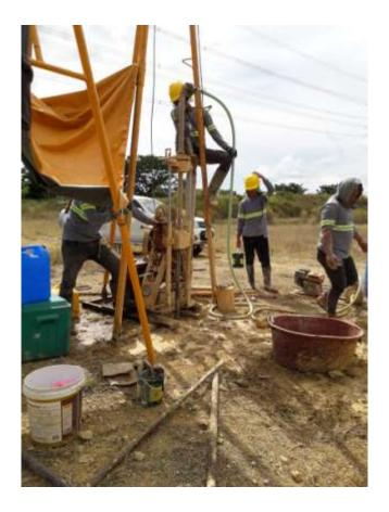
Ongoing setting out and soil investigation work for the new 12km Transmission Line
