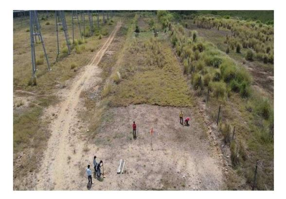
Initial tower foundations completed for the new 12km Transmission Line
