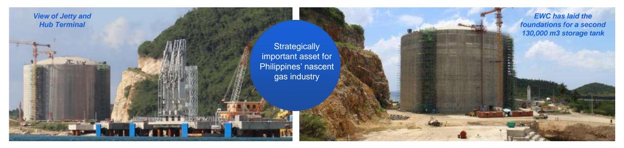
130,000 m<sup>3</sup> LNG Hub Terminal is 90% completed Deep water jetty is capable of handling all sizes of LNG vessels Facility can handle a throughput of 3 MTPA of LNG with the 1st tank, which can support 3,000 MW of gas fired power generation This will support our adjacent 650 MW combined cycle gas fired power plant, and provide expansion options for both EWC and third party gas clients Hub Terminal to be run on a tolling model for third party clients
