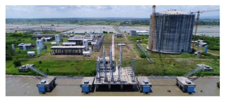
The Sengkang LNG Plant has a design capacity of 2 mtpa, consisting of 4 modular 500,000 tpa trains, an import/export and jetty facilities. Construction is 80% complete, having been delayed since 2017 due to land zoning claims which have since been fully resolved. Remobilisation work has commenced at site.
