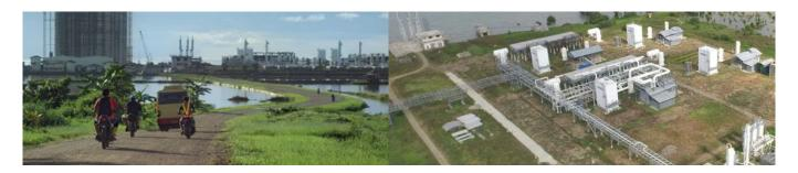
The Sengkang LNG Plant has a design capacity of 2 mtpa, consisting of 4 modular 500,000 tpa trains, an import/export and jetty facilities. Construction is 80% complete, having been delayed since 2017 due to land zoning claims which have since been fully resolved.
