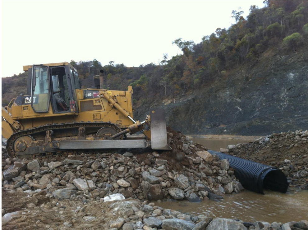
Figure 3: Construction of the river crossing to provide access to the east side of the Imaloto River
