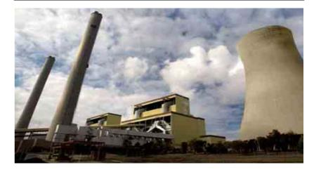
LYA power plant is a four unit 2,195MW brown coal steam turbine power station, integrated with an adjacent mine with reserves sufficient for at least 50 years
